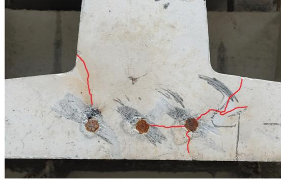
**Figure 3.** Actual cases of reentrant corner crack formation.
