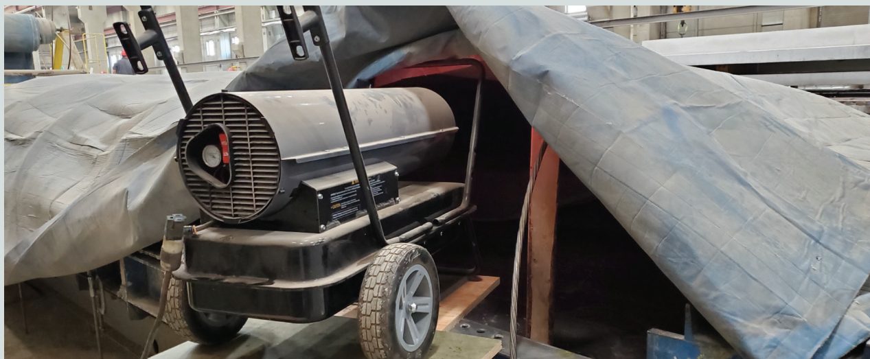
Figure 3. One supplemental forced-air heater, shown here, was placed at each end of the casting bed during portland cement concrete beam curing.
