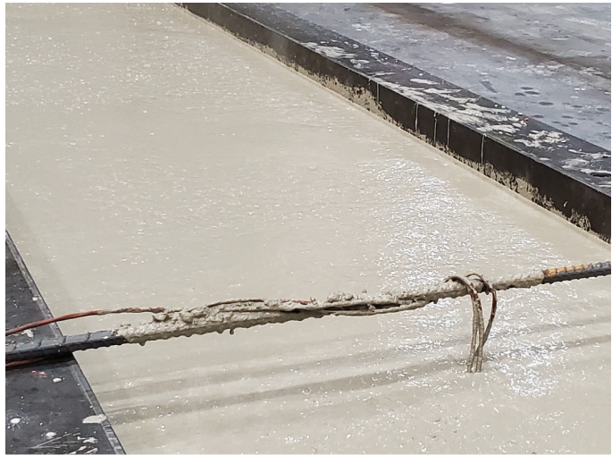
Portland cement concrete
