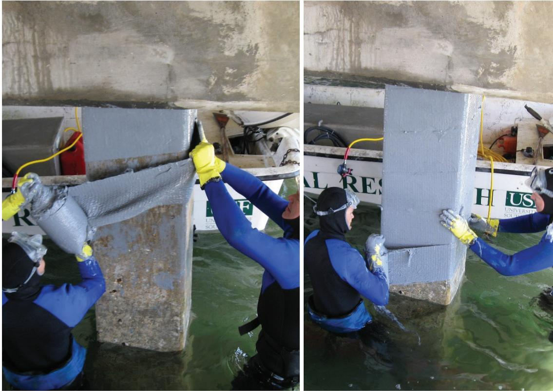
**Figure 2.** Fiber-reinforced polymer confinement applied from cap to mudline to arrest corrosion-induced crack growth.
