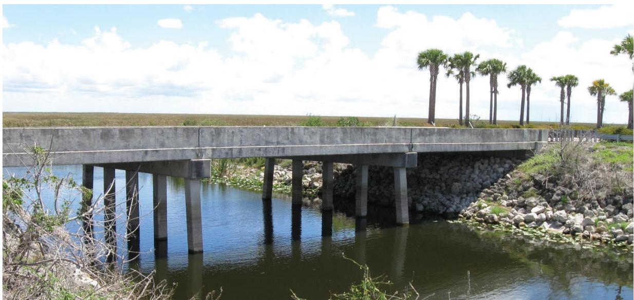
**Figure 1.** Typical pile bent built in the 1970s. This example is from the Alligator Alley stretch of southbound Interstate 75 in southern Florida between Naples and Fort Lauderdale.
