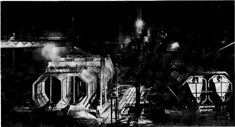
Fig. 4. Tunnel sections for Rotterdam Metro
