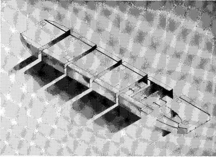
Fig. 3. Segmental construction of prestressed concrete barges (USSR)
