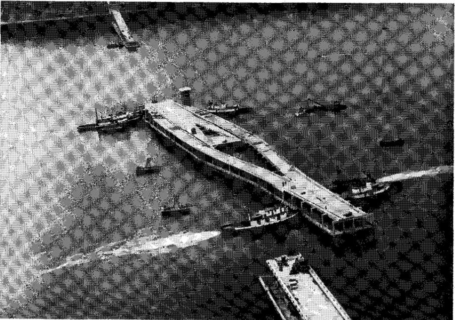
Fig. 2. Prestressed concrete floating bridge, Hood Canal, State of Washington. March-April 1971
