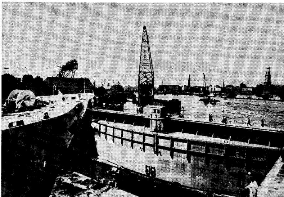
Fig. 1. Prestressed concrete dry dock caisson gate at Hamburg, Germany
