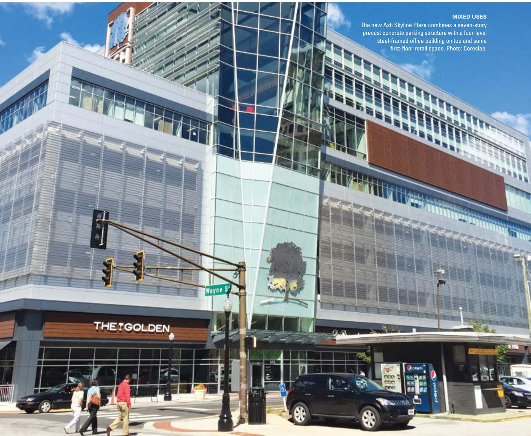
that, the west elevation features an architectural precast concrete fire-separation wall that was designed to be load bearing to accept tees when the project moves ahead.
