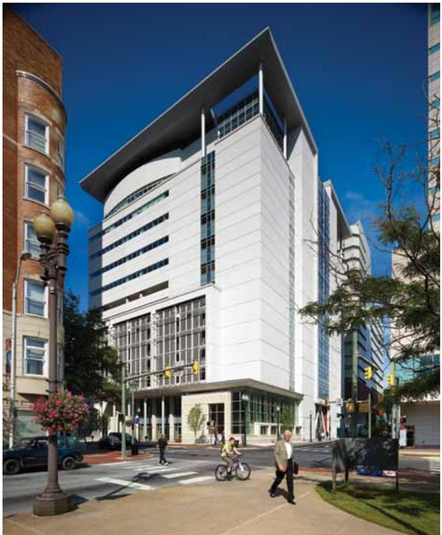
*The new 16-story academic building at the Harrisburg University of Science & Technology features architectural precast concrete panels on its exterior and a total-precast concrete parking structure. The building features a 125-seat auditorium and outdoor roof gardens. The campus is entirely new and consists of four sectors: this academic center as well as a business incubator, student village, and corporate-office complex.*
