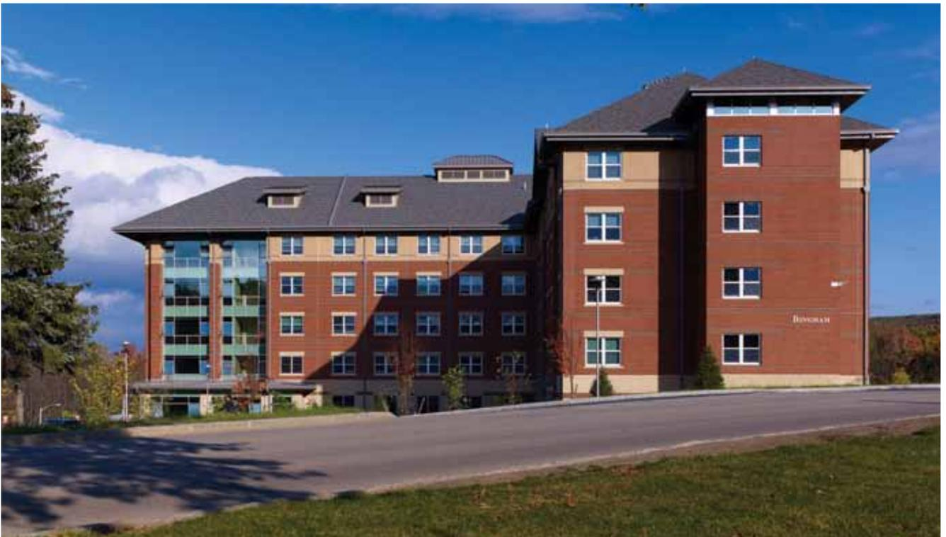
*The East Campus Housing facility at SUNY in Binghamton, N.Y., consists of four residential halls making up the new Dickinson Community. The dorms will be clad with architectural precast concrete panels embedded with thin brick to blend with other campus structures. The work is expected to be completed by the fall of 2013.*
