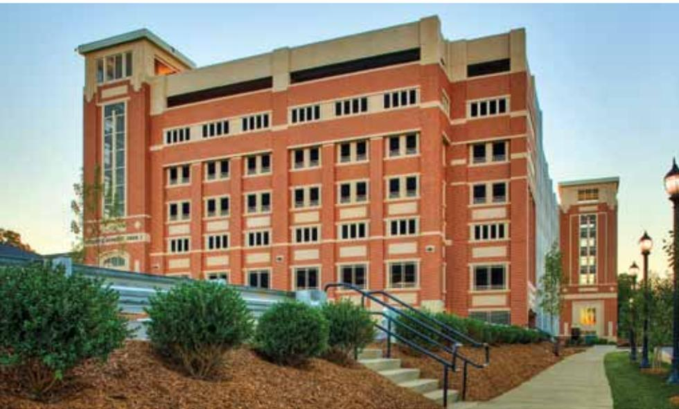
The new eight-level, 1,002-car parking structure at Central Piedmont Community College features a total-precast concrete structural solution. Two concrete pigments, one between bricks and one on larger portions, sometimes in the same panels, were used to achieve the appearance that the designers sought.
