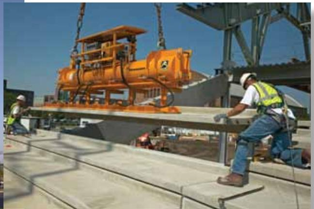
*A specialized vacuum-clamp lifting device allowed the large structural seating components to more easily be transported and rotated as needed throughout the construction process. Photo: Steven Bergerson*
