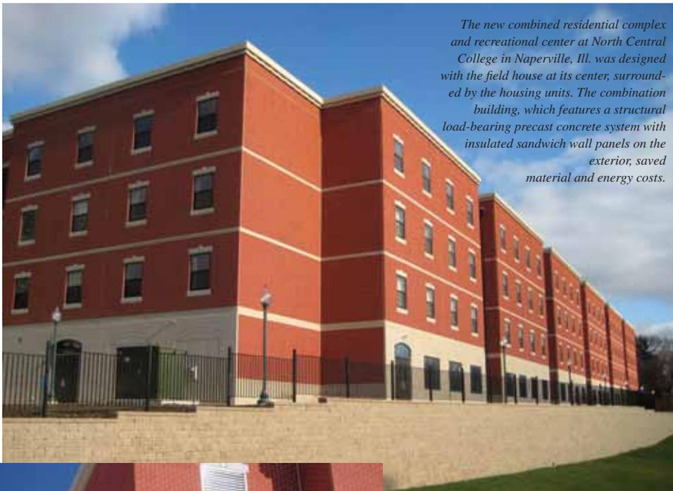
The new combined residential complex and recreational center at North Central College in Naperville, Ill. was designed with the field house at its center, surrounded by the housing units. The combination building, which features a structural load-bearing precast concrete system with insulated sandwich wall panels on the exterior, saved material and energy costs.
