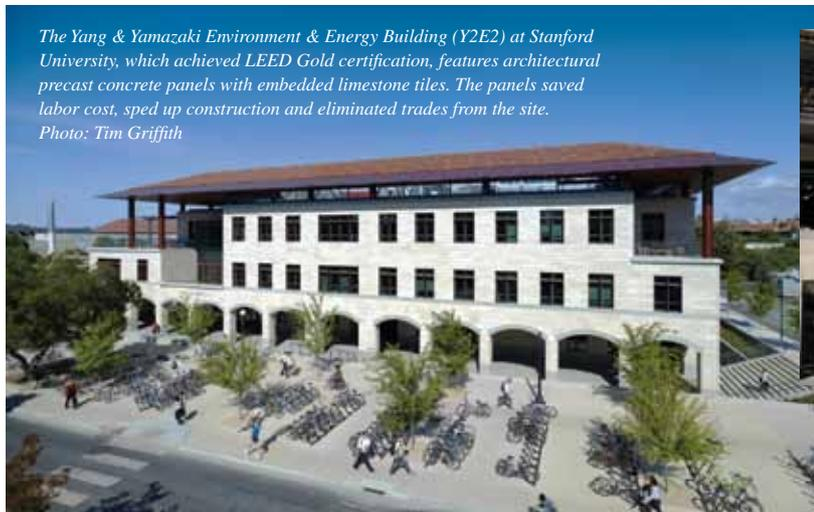
*The Yang & Yamazaki Environment & Energy Building (Y2E2) at Stanford University, which achieved LEED Gold certification, features architectural precast concrete panels with embedded limestone tiles. The panels saved labor cost, sped up construction and eliminated trades from the site. Photo: Tim Griffith*
