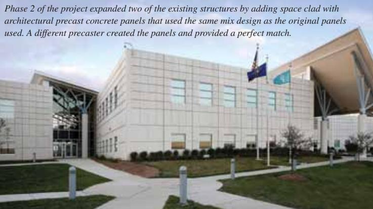
Phase 2 of the project expanded two of the existing structures by adding space clad with architectural precast concrete panels that used the same mix design as the original panels used. A different precaster created the panels and provided a perfect match.
