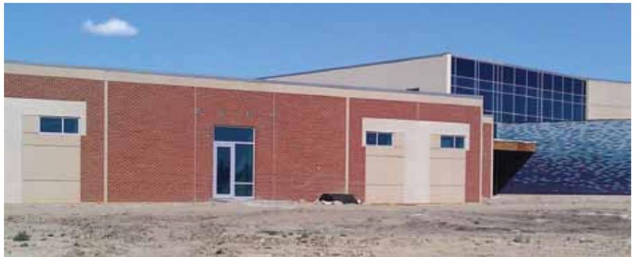
This 57,862-square-foot K-5 school uses precast concrete insulated sandwich wall panels to help meet its program requirements. The combination of three finishes on the exterior walls creates a unique look that helps the school blend into its surroundings.
