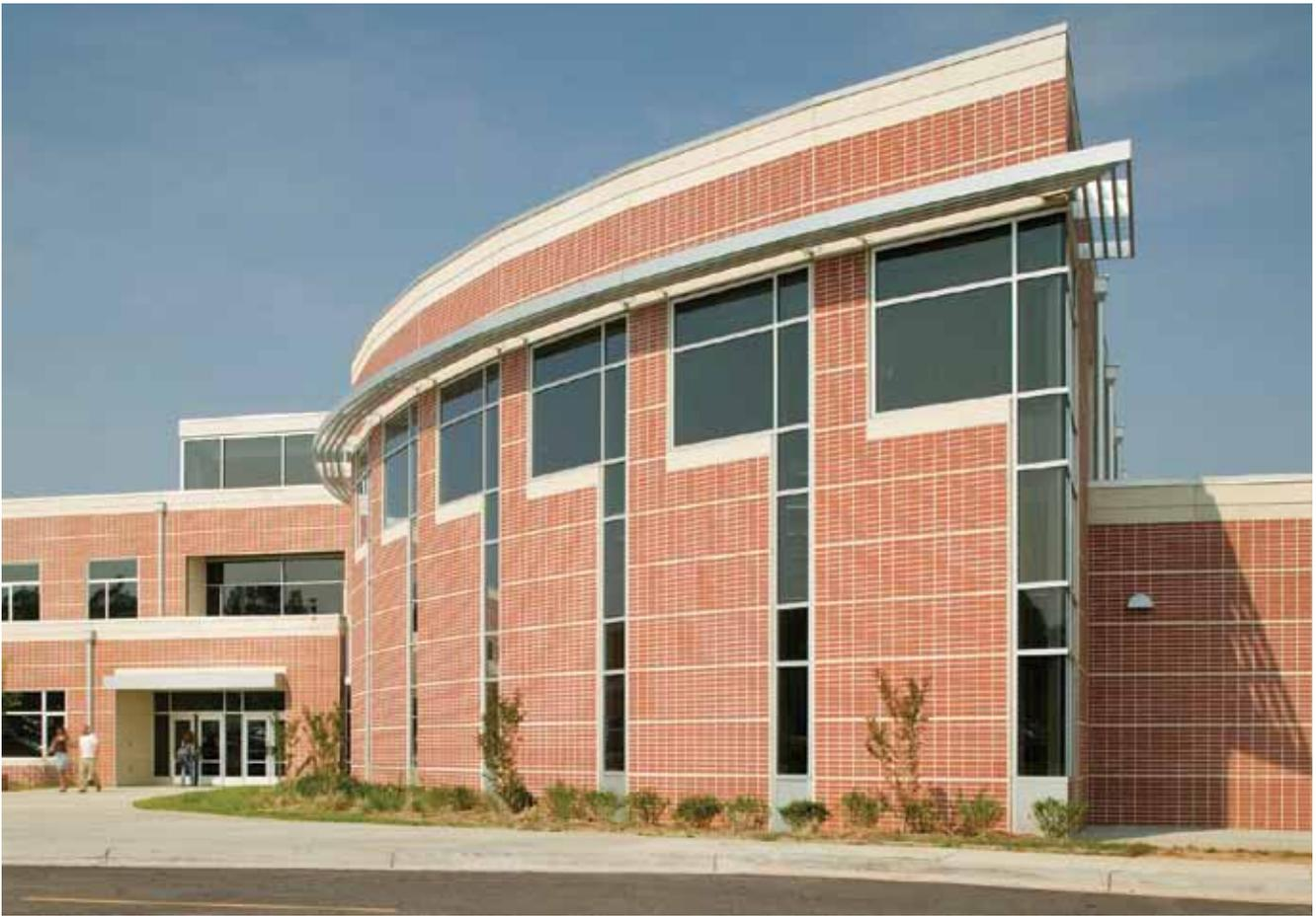
*Travelers Rest High School in Travelers Rest, South Carolina, welcomes students with an exterior featuring precast concrete exterior wall panels accented with thin brick. Photo: Perkins+Will*
