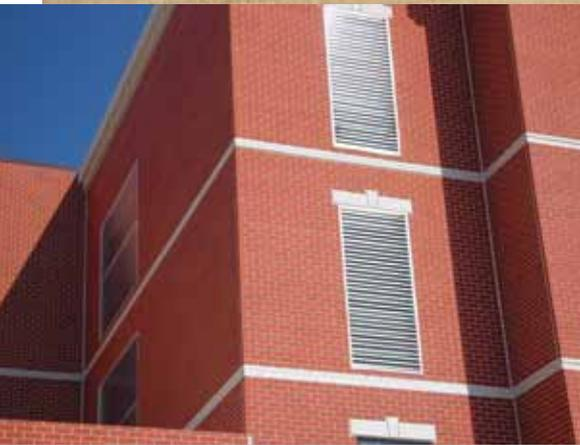
The panels' exterior appearance was achieved with formliners, each of which was used for 84 pours, cutting costs with the repetition.
