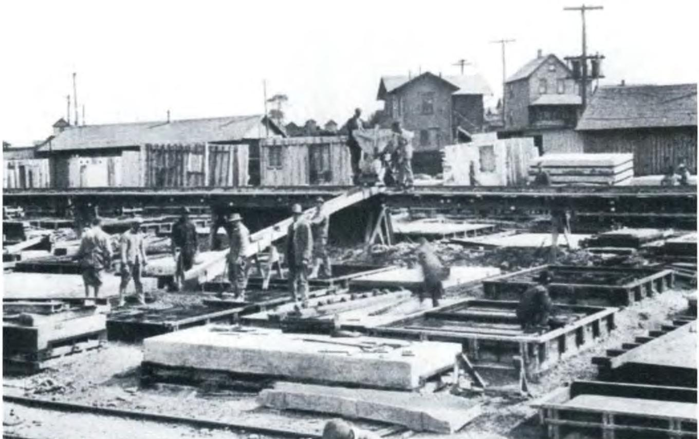
Fig. 2. An early precast concrete housing project in Youngstown, Ohio, included 281 units built between 1916 and 1920. A trestle track ran from the central mixing plant through the casting yard. Here concrete is being chuted from a sidegate car on the track into wood or concrete forms.
