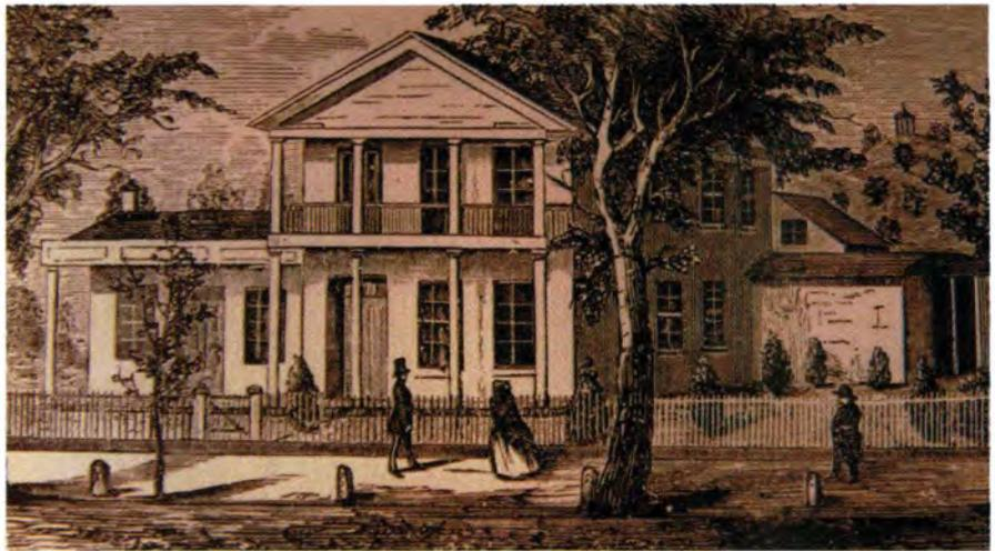
Fig. 1. *The Poor Man's Home and the Rich Man's Palace* was the title of a book George Barrett published in 1854 to describe construction of this concrete house in Spring Valley, Ohio. The sand, gravel, and lime mix was supplemented in some places with cobblestones to speed filling of the forms.
