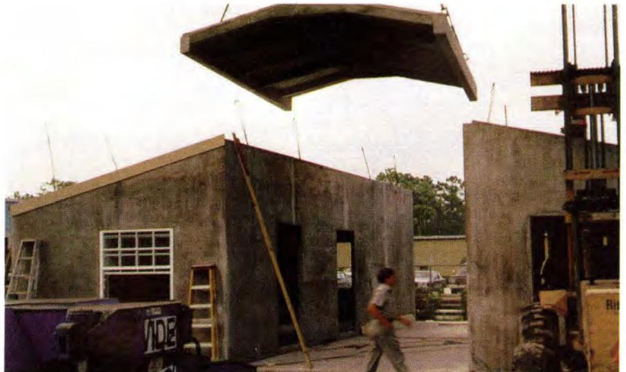
Fig. 7D. With two box modules in place on the slab, precast roof is being lowered into position.
