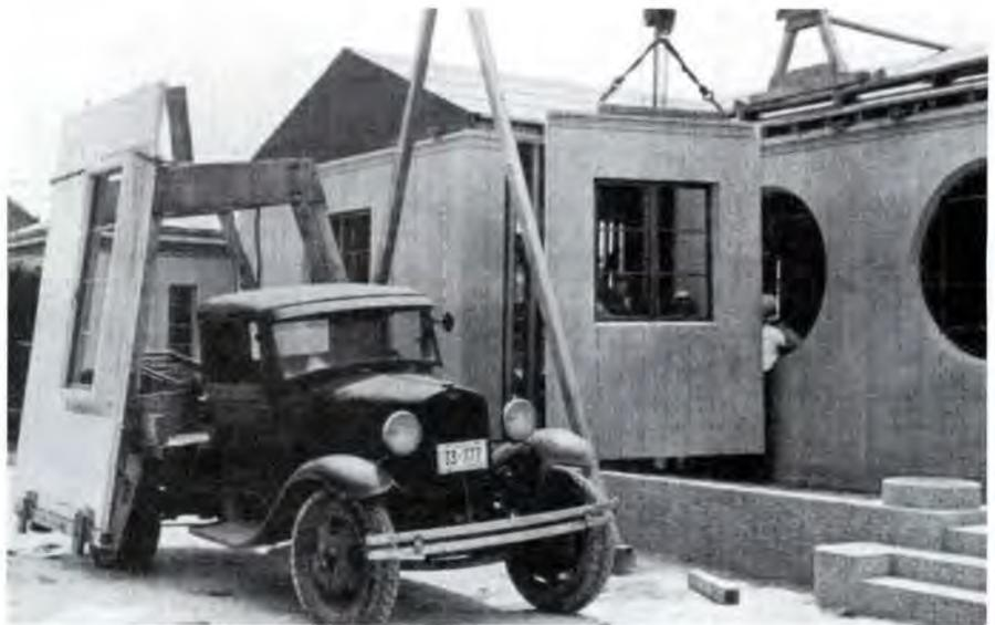
Fig. 3A. Erecting the walls of one of the Colesville Pike precast concrete houses, Silver Spring, Maryland, 1935. The completed Polychrome House is visible in the background (Courtesy: Reni Photographers).
