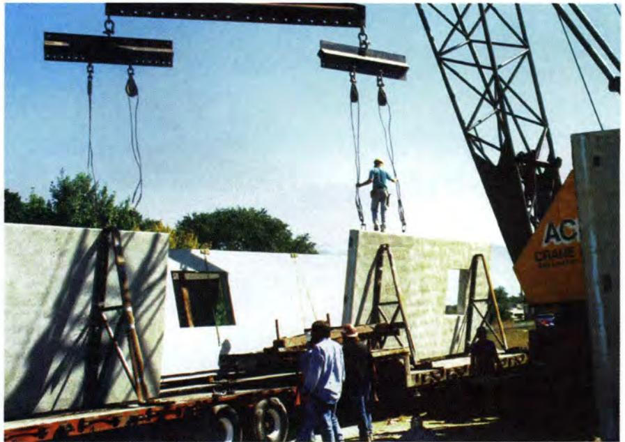
Fig. 9A. Sandwich panels trucked to the site are lifted by crane for assembly of a home.
