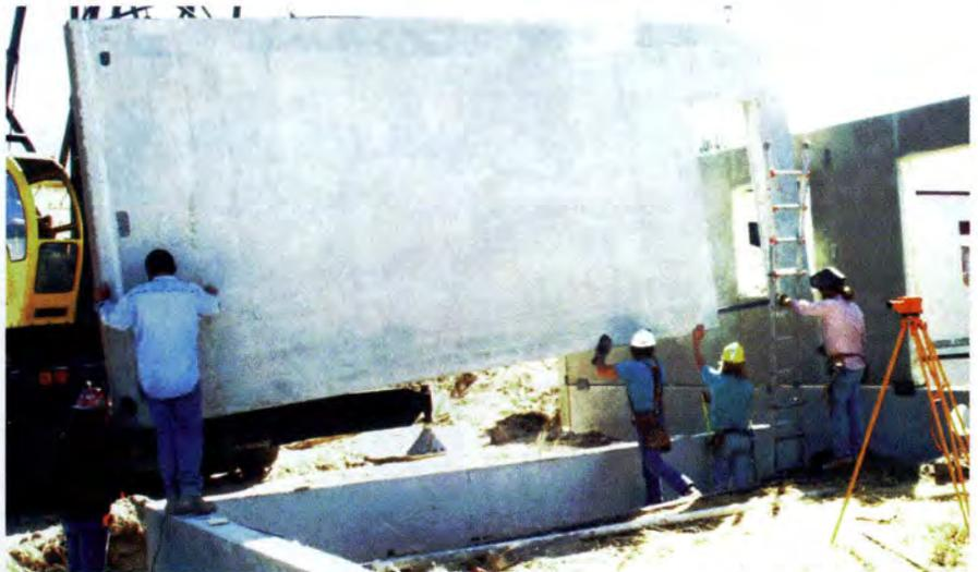
Fig. 9B. Workers guide panel into position on precast foundation wall.
