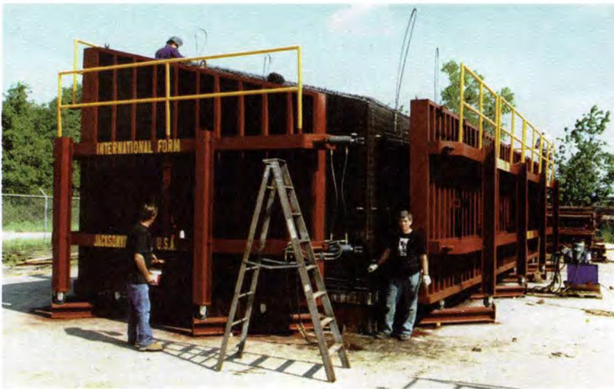
Fig. 7A. Sloping roof is part of the five-sided precast module cast in this hydraulically operated form.
