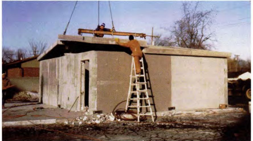
Fig. 10A. Prototype structure being erected with site-cast laminated panels. Precast panel used for sloping roof.
