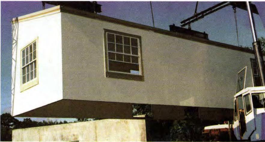
Fig. 7B. The box module ready for placement on a slab has been coated and sealed, with windows installed.
