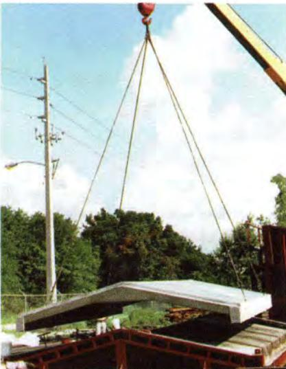
Fig. 7C. Precast concrete roof module being lifted from its form.
