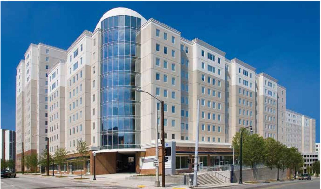
*Georgia State's University Commons 2000-bed residential hall features insulated precast concrete wall panels that provided a strong, permanent appearance, allowed the building to be completed earlier than scheduled, saved \$1 million in construction costs and maximized energy savings over the building's life. All photos courtesy of Metromont Corp..*
