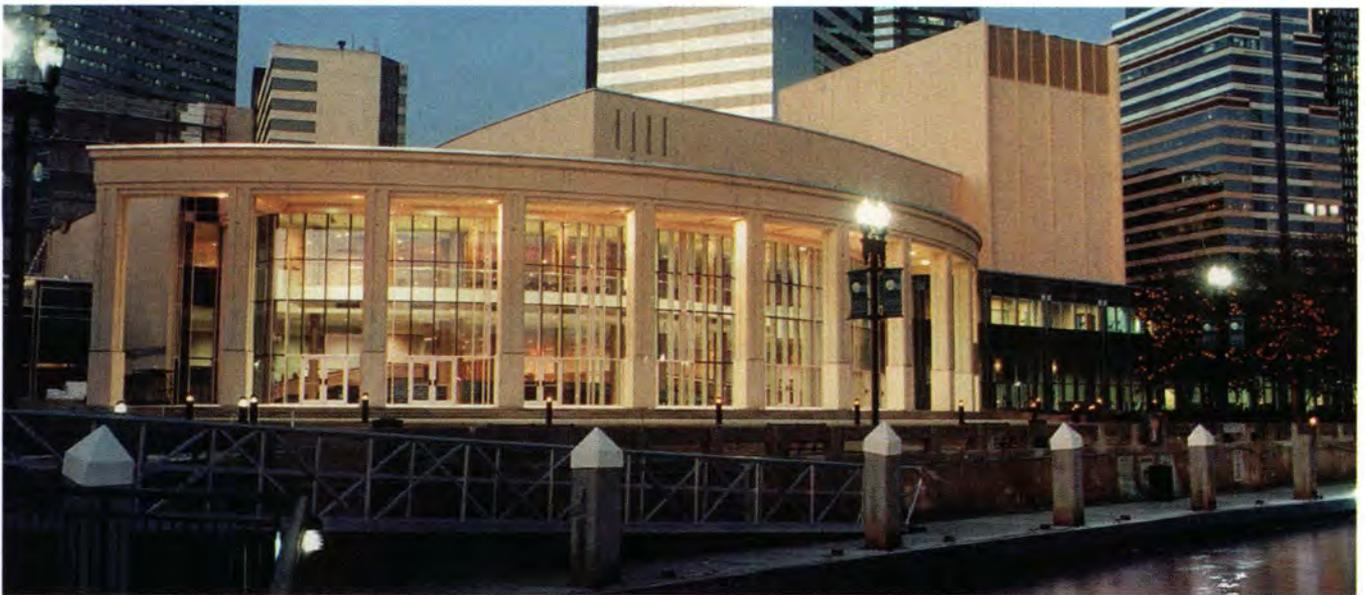
Fig. 1. The new \$32 million Times-Union Center for the Performing Arts in Jacksonville, Florida, includes a \$10.6 million concert hall (foreground) consisting of an all-precast concrete structure, including loadbearing acoustical walls for the theater.
