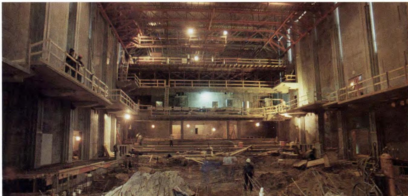
Fig. 8. Using precast concrete panels allowed the new theater to be enclosed much faster than would have been possible with other systems. It also provided the strength and thin profiles required to add two balconies into the space and reach the necessary seating requirement.
