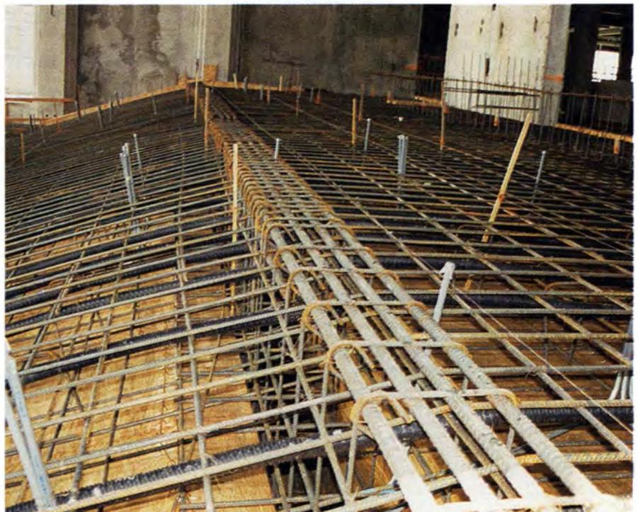
Fig. 12. Post-tensioning tendons and mild steel reinforcement for balconies.
