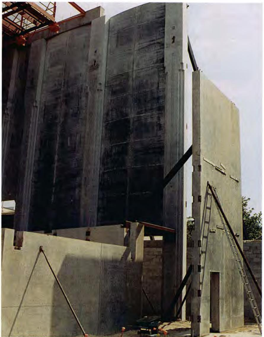
Fig. 9. The precast structure comprises a variety of components, including loadbearing panels that were curved on the interior for proper acoustics and flat on the exterior. These exterior walls were furred out and clad with drywall to serve as the corridor outside the theater.
