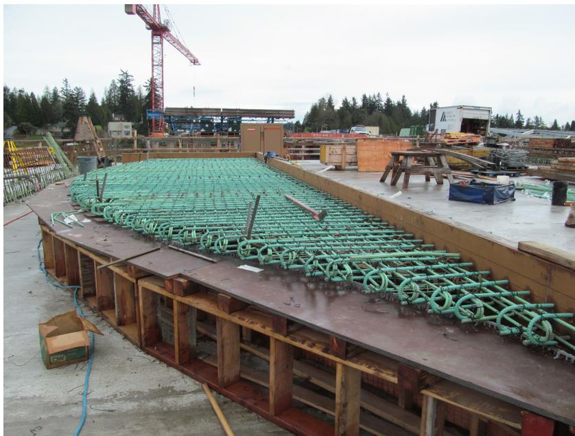
**Figure 18 - Rebar and formwork assembled on the bridge deck getting ready to cast the belvedere.**
