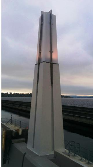
**Figure 24 - Minor element with precast concrete base and stainless steel translucent panel fixture.**
