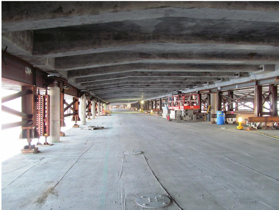
**Figure 12 - The ribbed deck panel soffit in the low-rise section.**
