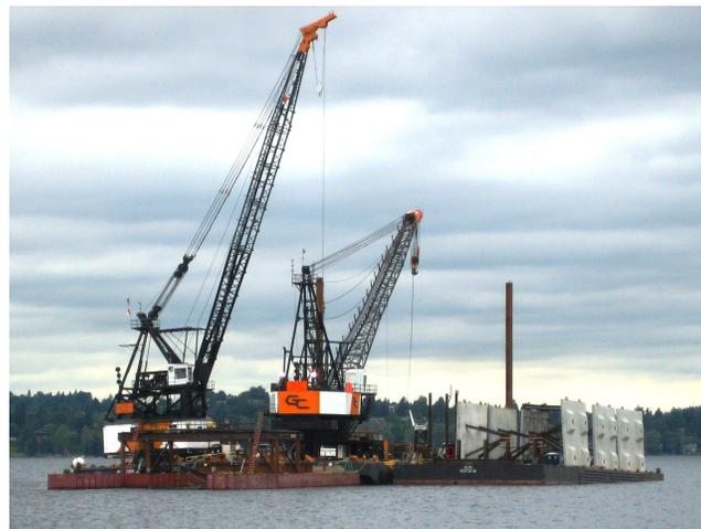
**Figure 10 - Fluke anchors being installed.**
