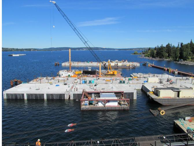
**Figure 9 - Pontoons being connected at the bridge site on Lake Washington.**
