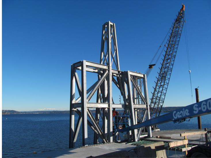
Figure 22 - Sentinel steel framing to support the precast cladding, as seen at the roadway deck.
