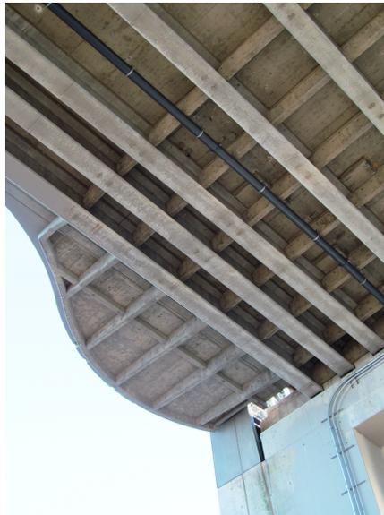
**Figure 20 - Soffit of the belvedere with the additional girder and ribs.**
