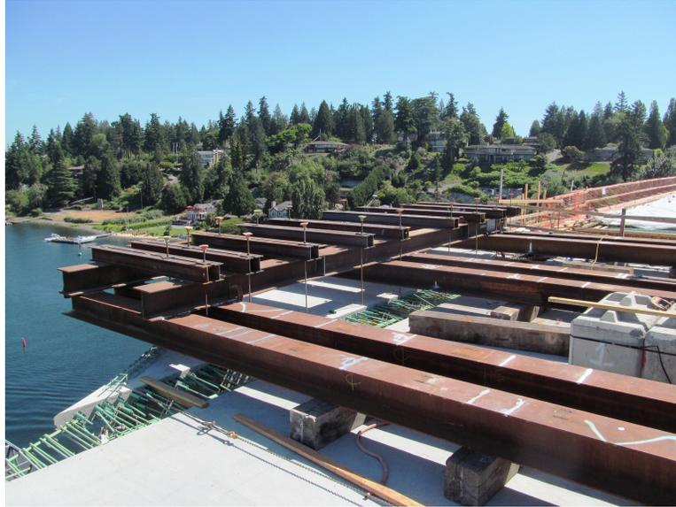
**Figure 19 - Steel false work supporting the precast belvedere while the closure pour and post-tension is installed.**
