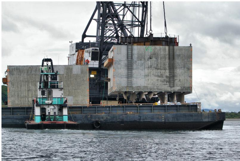
Figure 11 - Gravity anchor being lifted from the barge to be set in the water in Puget Sound.
