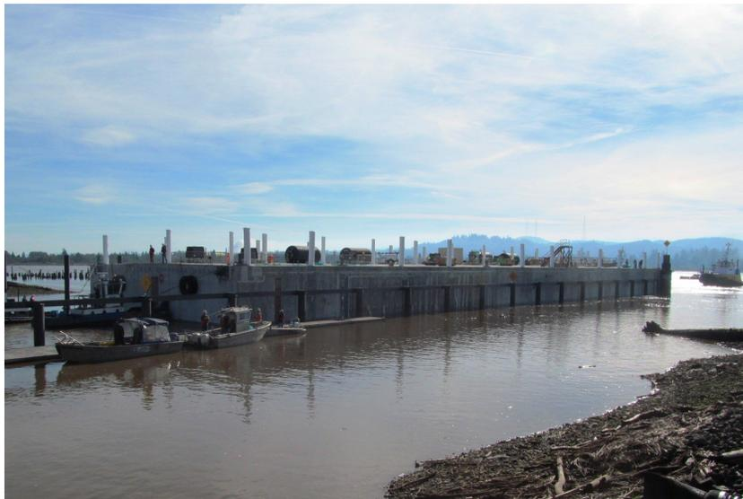
**Figure 8 - A longitudinal pontoons being floated out from the casting basin in Aberdeen, WA.**
