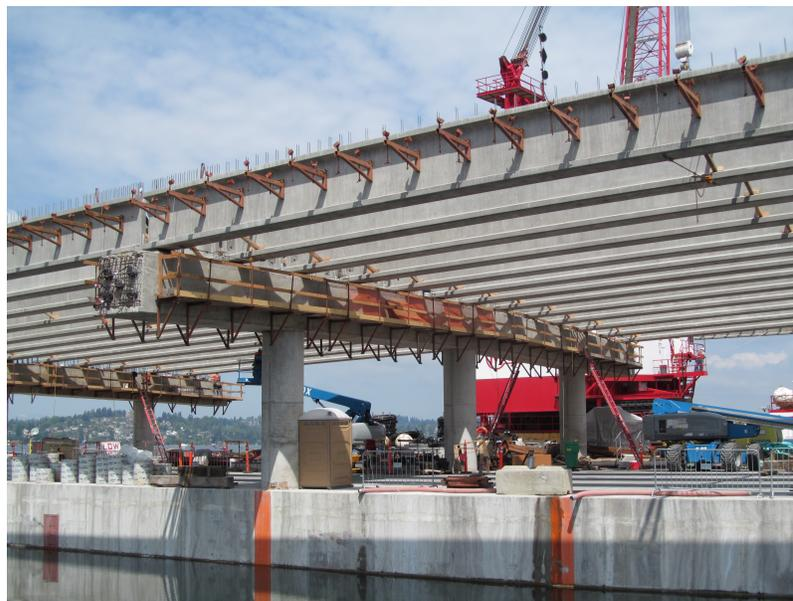
**Figure 17 - Precast girders set on a west high-rise post-tensioned cantilever crossbeam.**
