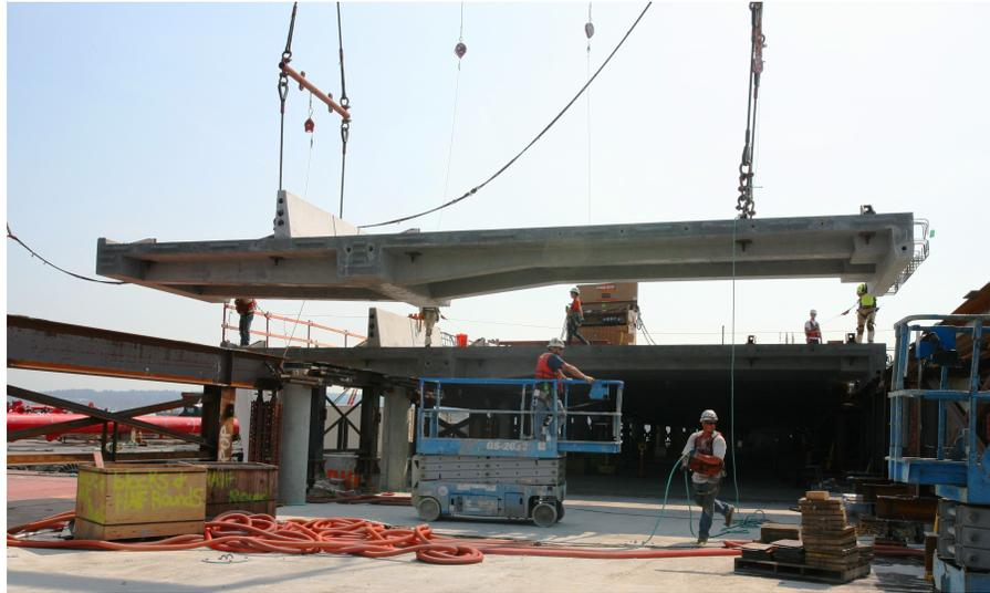
**Figure 13 - Setting a low-rise panel on the false work.**
