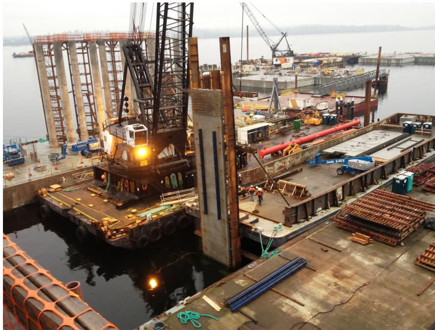
**Figure 15 - Pontoon W precast box column panel being tilt vertically.**
