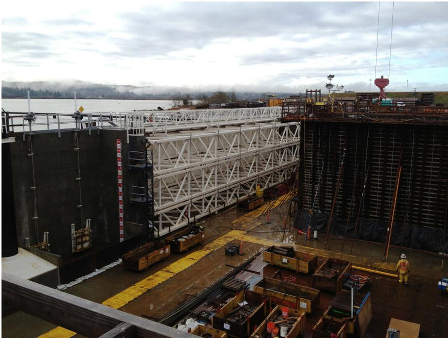
**Figure 6 -The white truss is the flood gate for the casting basin in Aberdeen, WA. On the left is a pontoon being constructed.**
