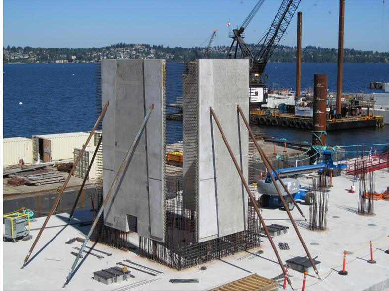
**Figure 16 - Pontoon A precast box column panels being erected.**
