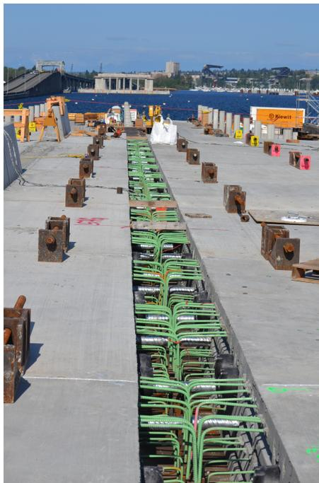
**Figure 14 - Temporary bars holding panels in place while the center longitudinal closure pour is constructed.**
