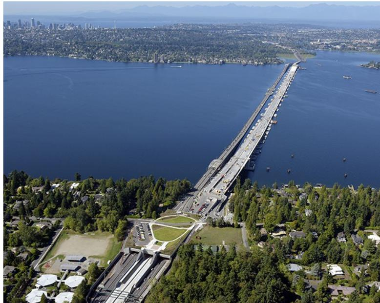
Figure 1 - The new SR520 Floating Bridge nearing completion, adjacent the original bridge.
