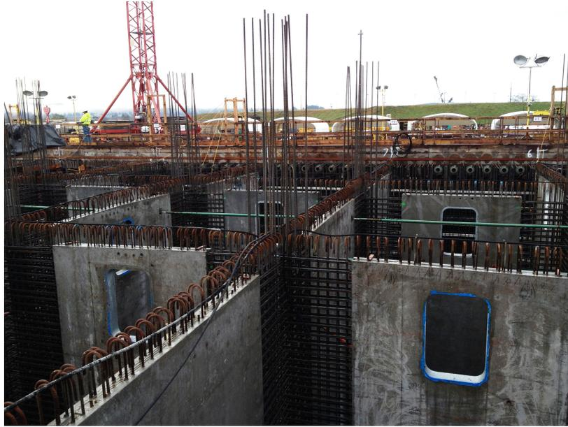
**Figure 7 - Precast interior wall panels erected in pontoon formwork. Joints between panels would then be cast. At the rear are the post-tension anchor heads.**
