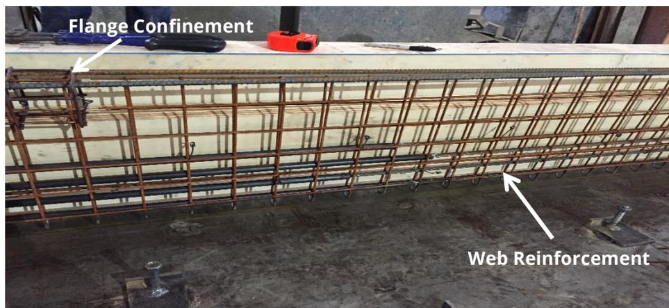
**Figure 4. WWF Reinforcement**
