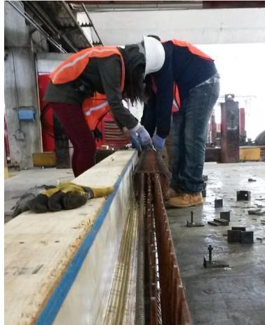
**Figure 7. Assembling the WWF Reinforcement**
