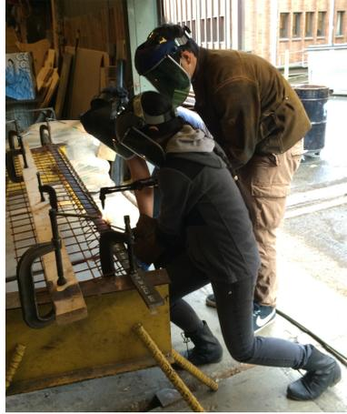
**Figure 6. Hot-Bending the Top Flange Confinement**
