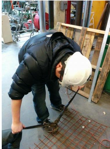
**Figure 5. Cutting the WWF**
