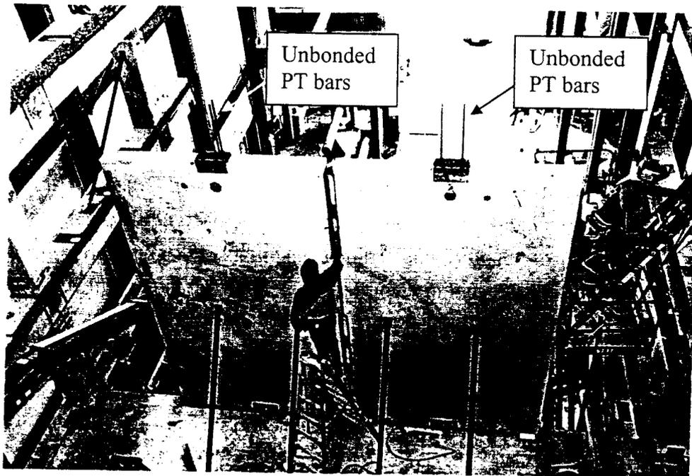
Figure 3.1 Construction of the jointed wall panel system.
