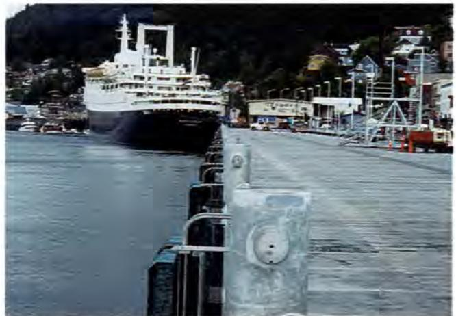
Fig. A. Typical precast, prestressed concrete grouted dock deck, Ketchikan, Alaska.
