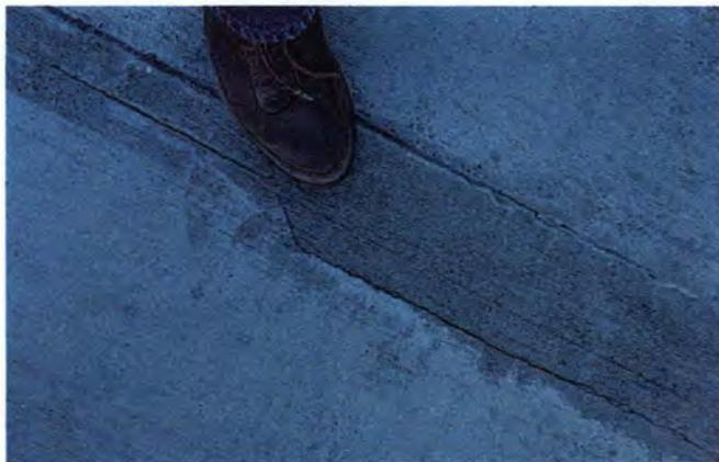
Fig. E. Portland cement based grout joint.
