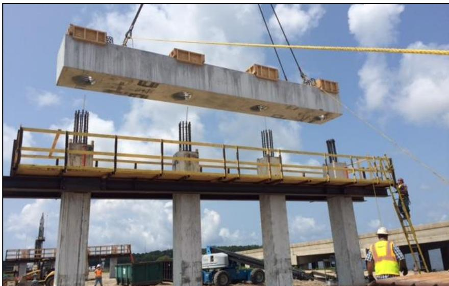
**Figure 13 – Setting Precast Bent Cap**
