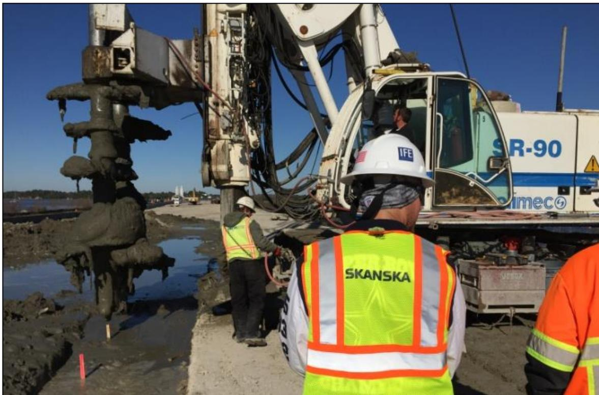
**Figure 11 – Soil Mixing**
