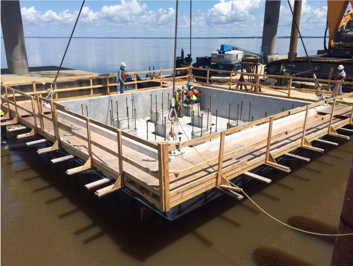
**Figure 10 – Precast “Bathtub” Footing Form**
