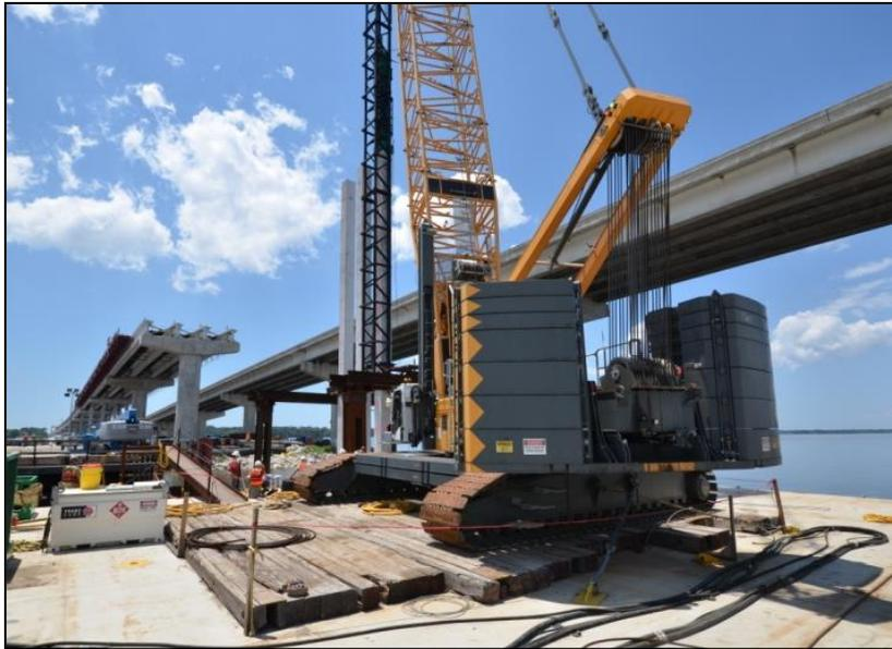
**Figure 12 – Pile Driving**
