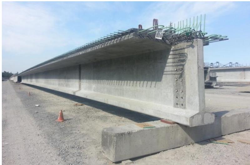
Fig. 2 Decked Bulb Tee Girder for Skagit River Bridge in Storage
