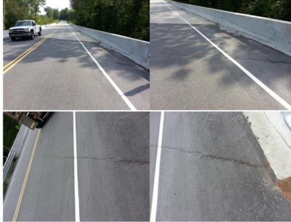
Fig.17 Photographs of observed cracks at approach slab/roadway interface
