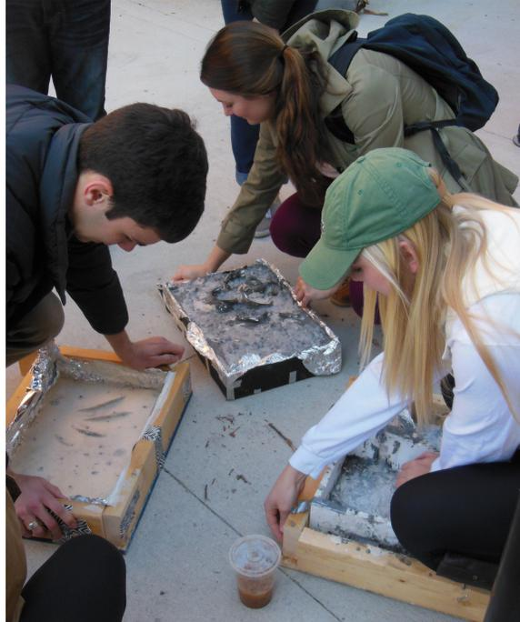
Fig. 1 Architecture students at Miami University working to release precast concrete panels from their formwork.
