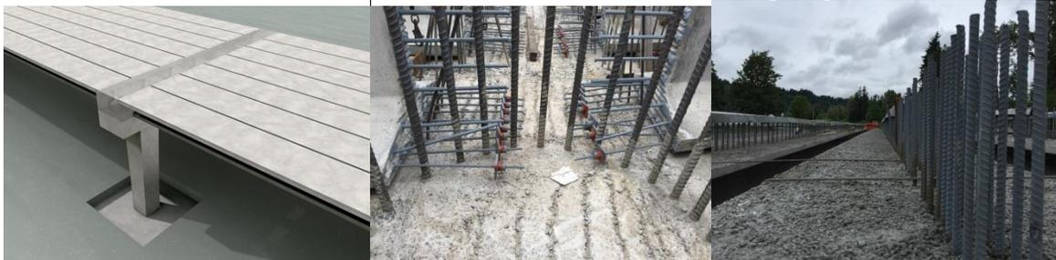
Figure 6. Semi-raised fixed integral diaphragm
