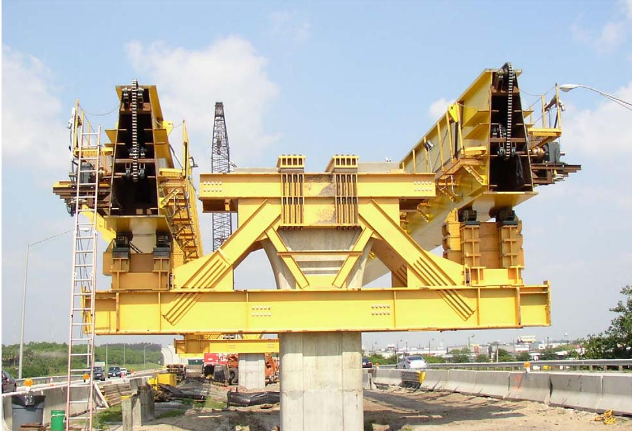
**Photo 1: Pier Bracket and Erection Girders**
