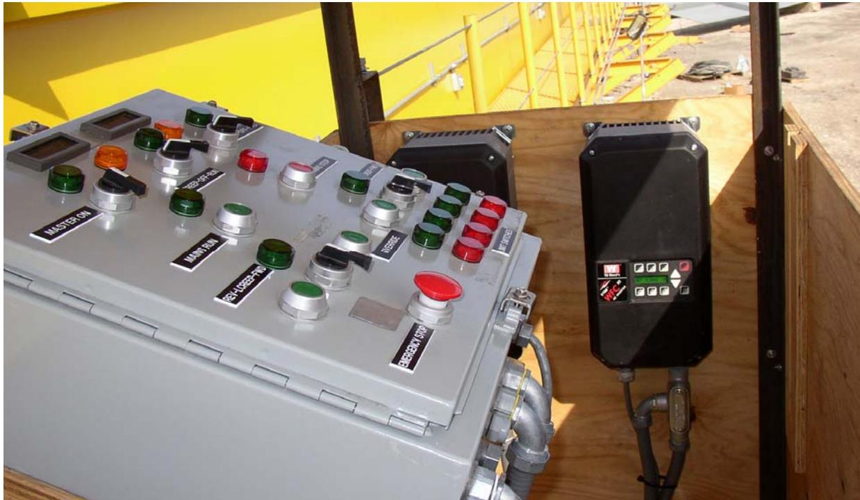
**Photo 3: Control Panel, Heading One, VFDs Behind**
