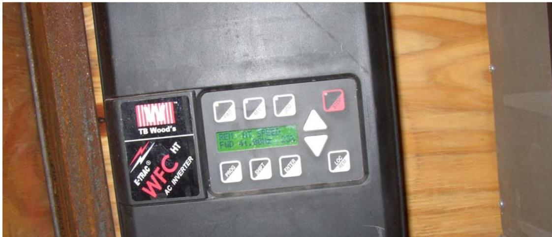
**Photo 6: VFD at Load, 41 HZ or 15 feet per minute
