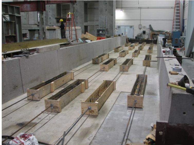
Fig. 5 Forms of the pullout specimens
