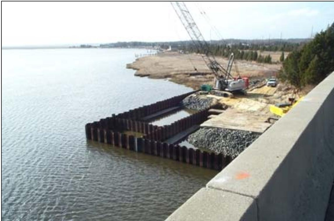
Figure 11 – Cofferdam for Demonstration Drilled Shaft and Pier 1
