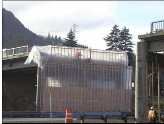
Fig. 9 Cold Weather Protection for Grout Pad Placement
