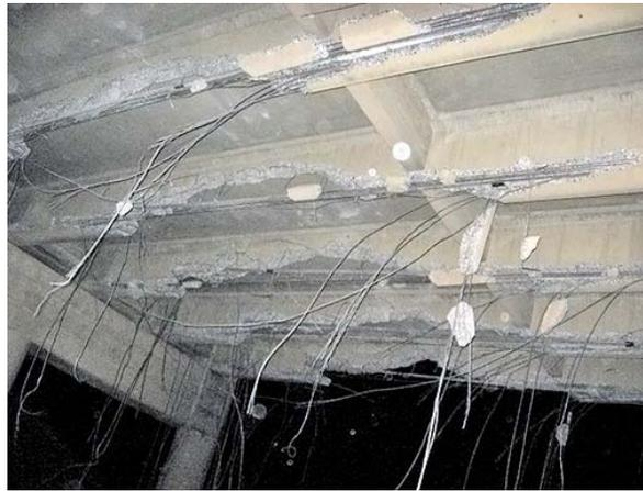
Fig. 5 Pipe Curvature Seen in Damaged Bridge Girders
