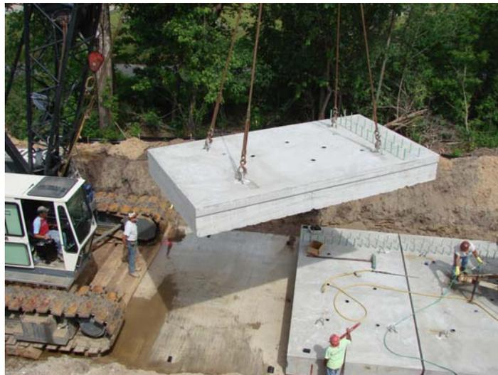
**Figure 9.** Erection of the Precast Footing Segments
