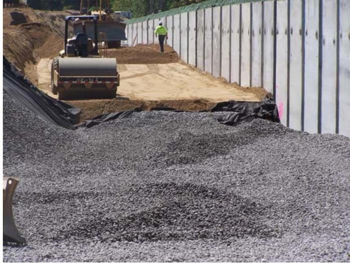
**Figure 14.** Structural Backfill and Light Weight Slag Placed behind the Walls.
