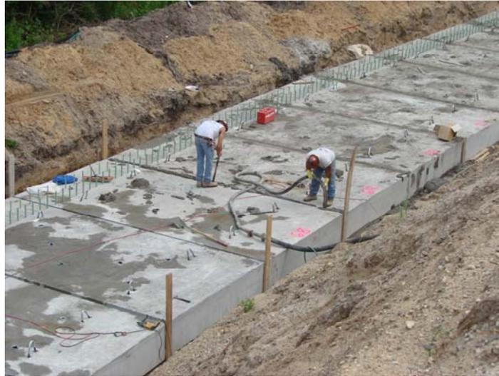
**Figure 10.** Grouting Operation for Footing Shear Keys
