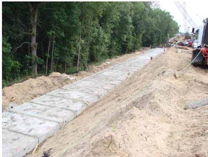
**Figure 11.** Erected Footing Segments of Wall A after Grouting
