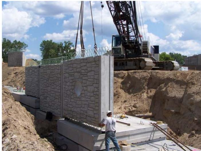
**Figure 12.** Erection of Short Stem Segments
