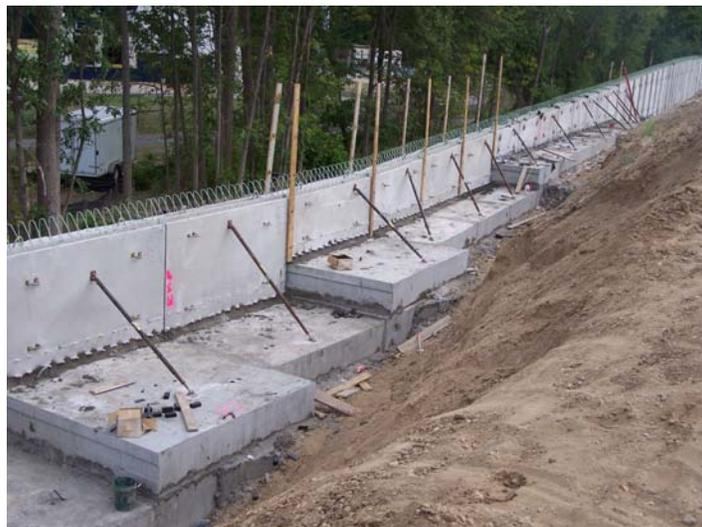
**Figure 13.** Bracing of Stem Segments
