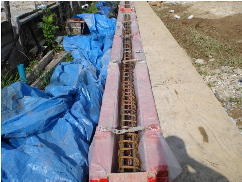
Fig. 1 Beam form and reinforcement cage before concrete placement
