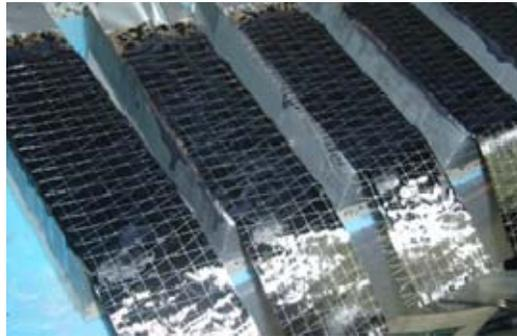
Fig.3: CF fabrics application by wet lay-up method
