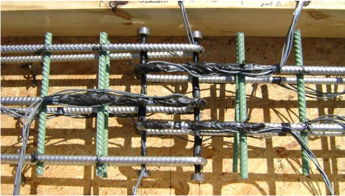
Figure 12: Stainless Steel Joint Detail (U-bar)
