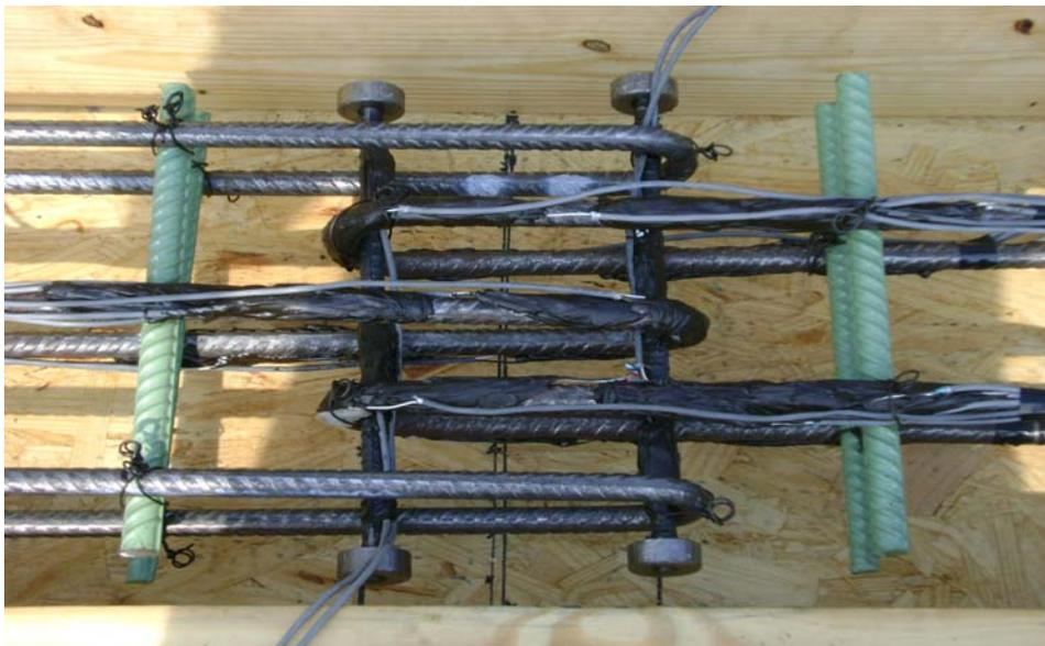
Figure 11: Welded Wire Reinforcement Joint Detail (U-bar)
