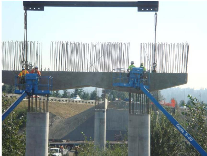
Fig. 8: Precast Bent Cap under Construction in Washington State
