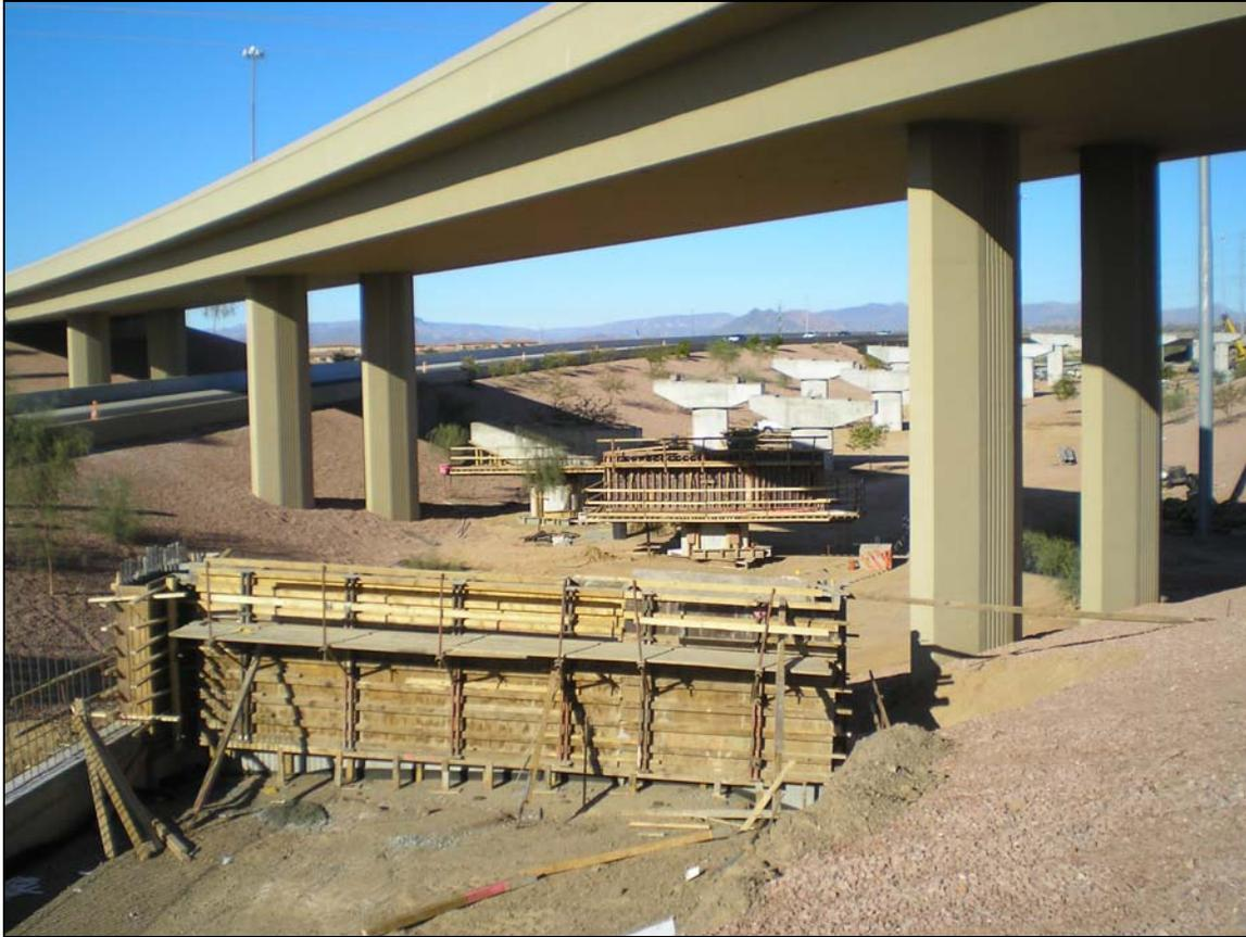
**Figure 06** – Looking northeast, abutment (foreground) and piers for dual bridges are staggered 38' for independent fine-tuned placement.
