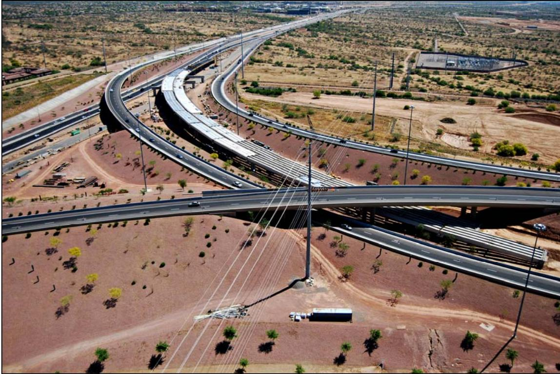
**Figure 05** – Looking east, dual bridges (separated by a 10” gap) carry HOV SB and HOV NB separately under Ramp NW, above the Reach 11 flood control basin, and over SR101L EB. Note, at left, SR101L EB is shifted to a detour and, at center, the overhead power lines’ constraints.
