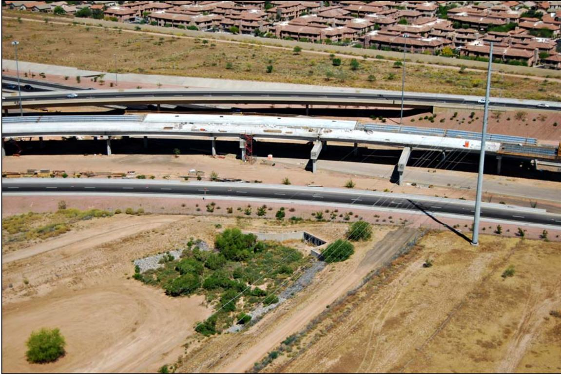
**Figure 08** – Looking north, the three straddle bents at (from LT to RT) Piers 10S, 10N, and 11N are level, zero-skew, and essentially identical. Additional constraints under and over SR101L are, at center, large RCBC (outlet visible) and, at right, overhead power lines.
