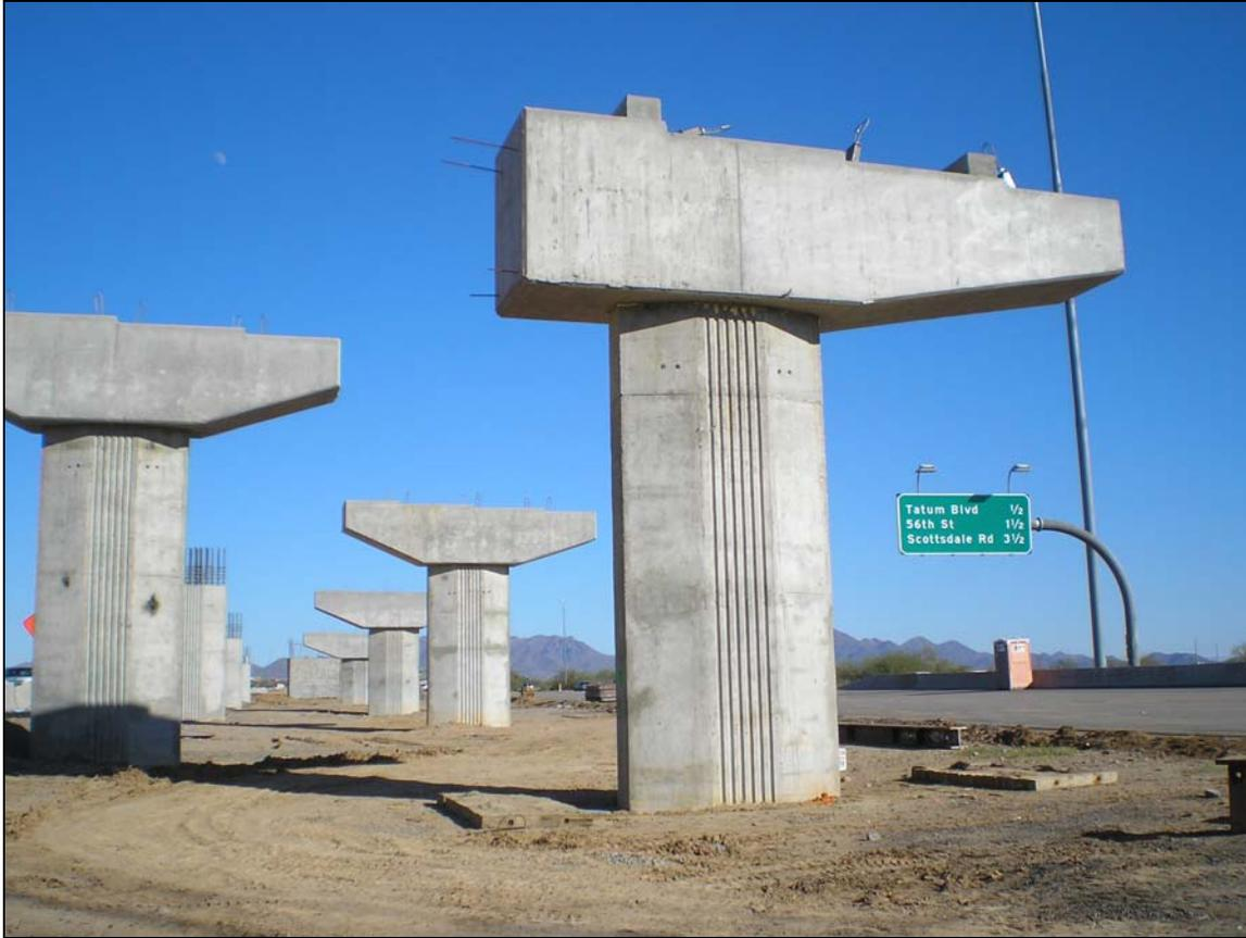
**Figure 12** – To clear an underground conflict, Pier 12N was redesigned as unbalanced cantilever to shift the drilled shaft and column.
