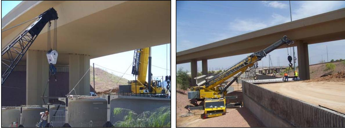
**Figures 14A and 14B** – Careful planning of pier locations proved invaluable for foundation drilling and girder setting. Shown are the two critical spans – at left looking south, is HOV SB Span 2 and, at right looking north, is HOV NB Span 1.
