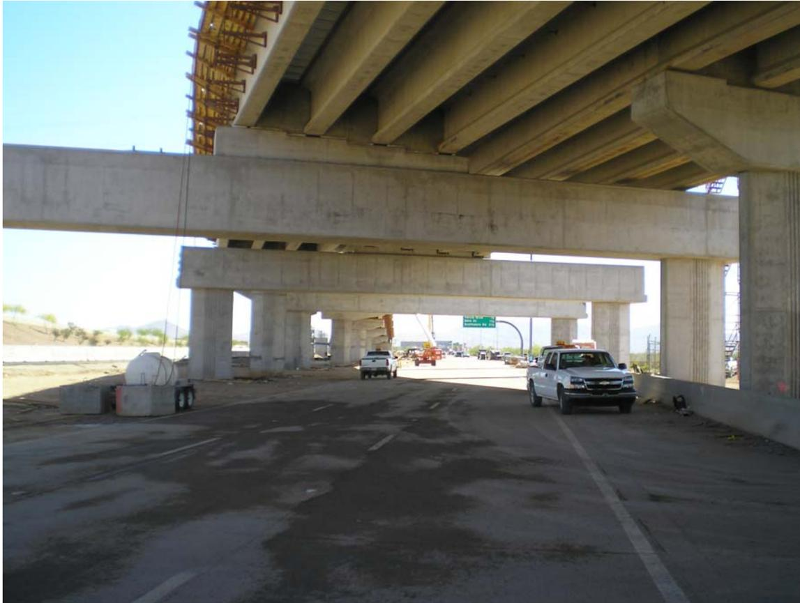
**Figure 01** – First of such applications in Arizona, straddle bents support only one-of-two bridges passing over them. Pedestals constructed atop the straddle bents transfer just one superstructure load to the substructure – the other superstructure does not touch. Straddle bent Pier 10S (foreground) carries the HOV SB Bridge (LT) – but not the HOV NB Bridge (RT); Pier 10N and Pier 11N (beyond) support only the HOV NB Bridge.
