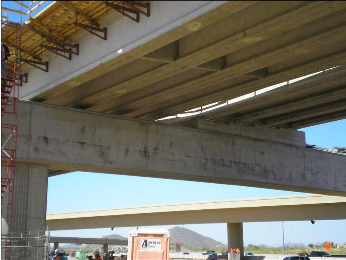
**Figure 11** – Looking west, straddle bent Pier 10S supports only the HOV SB Bridge (right) while the HOV NB Bridge (left) hurdles over, clear by about 8”.
