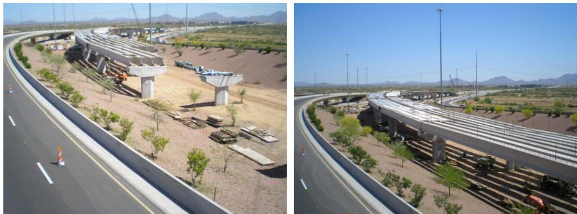
**Figures 16C and 16D** – First framing plan mobilization involves 84 girders (LT); and as deck construction has commenced, second mobilization involves 32 girders (RT).
