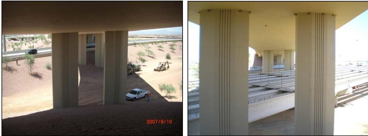
**Figure 07A and 07B** – Looking north, HOV SB and NB Bridges pass under the existing Ramp NW Bridge with limited headroom. Final Design bridge layouts move all piers and foundations out from under the shadow of the existing bridge.
