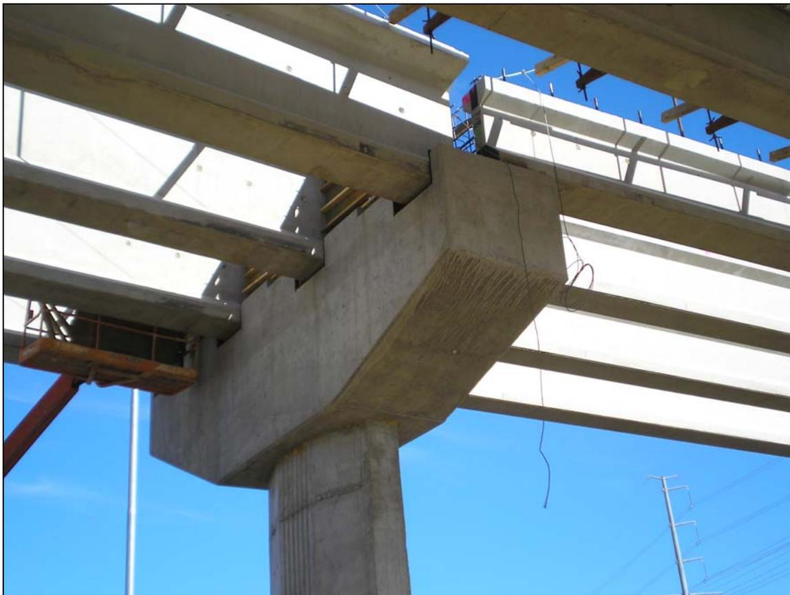
**Figure 10** – Where the 126' spans and 102' spans adjoin, beam pockets receive the bottom flanges of the deeper back-station girders. Hammerhead Pier 11S shown, pedestal for straddle bent Pier 10N similar.
