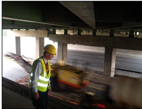
Fig. 1 Bridge in Georgia rehabilitated with steel pedestals to increase vertical clearance
