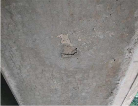
*Figure 9. Cracking at bottom of girder*
