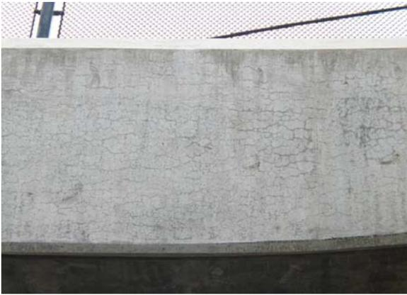
*Figure 10. Cracking in CIP girder*
