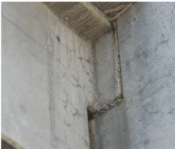
Figure 8. Cracking at girder end
