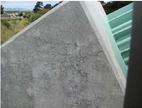
*Figure 11. Cracking in CIP anchorage*
