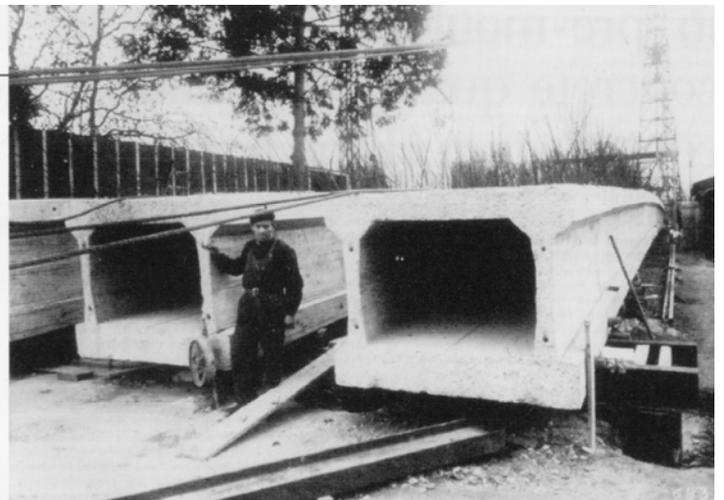
Figure 10 - Luzancy Bridge segment assembly
